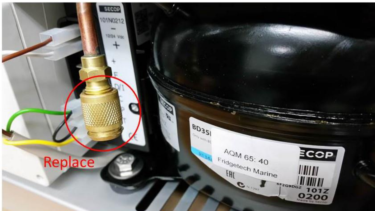
Figure 4-41 Replace the protection cap once you have finished the process
