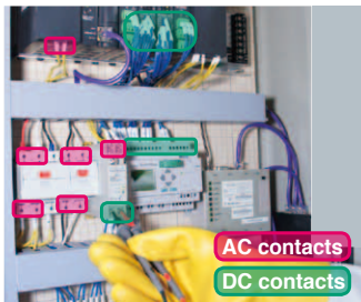
A mixture of AC and DC signals
