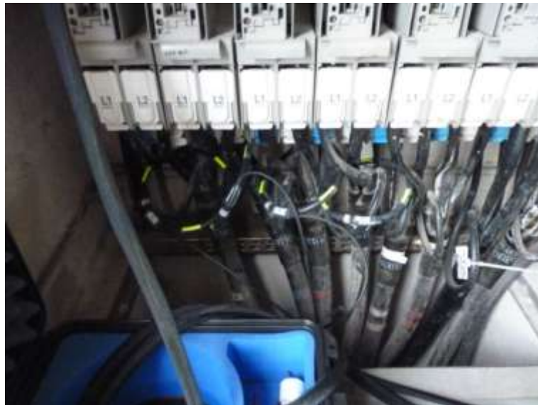
Figure 5 Installation of current coils around each TIPI feeder
