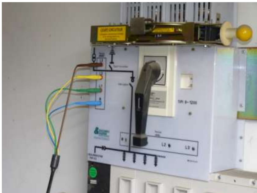
Figure 4 Voltage connection via \varnothing 4\text{mm} plugs from the TIPI voltage outputs
