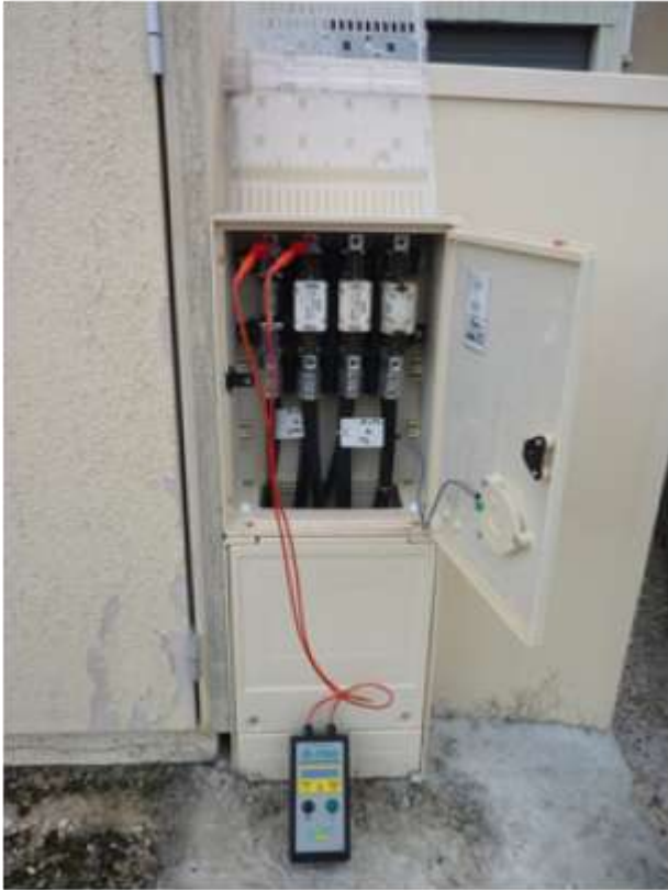
Figure 12 Connection by croc clips
