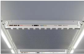
Clean room ceiling
